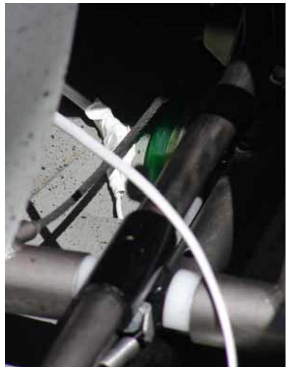
Cramped space for the cable into the nose
